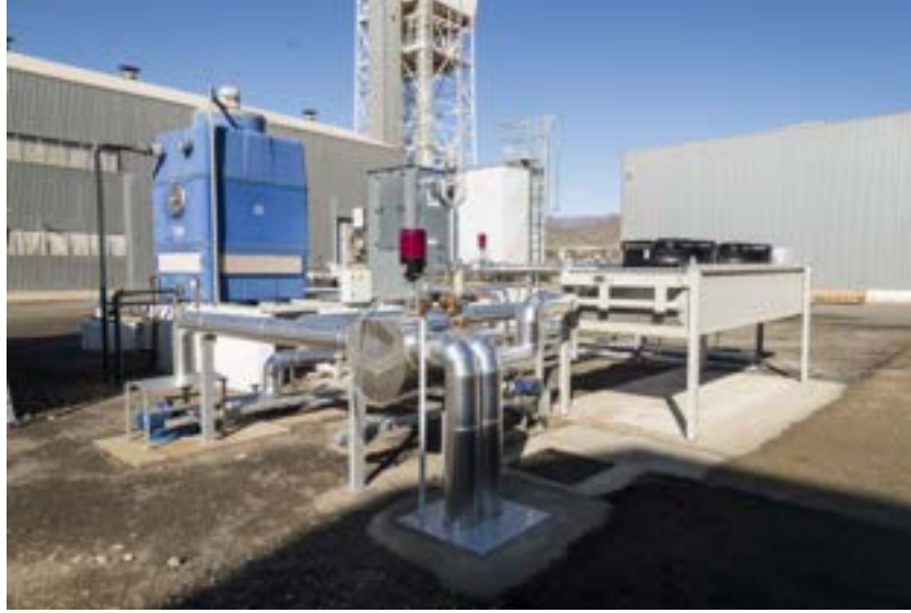
Figure 2: Picture of the cooling circuit in the combined cooling pilot plant at PSA.
